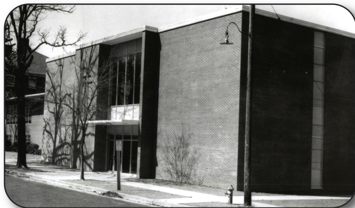
This is a view of the northeast side of the Hall & Auditorium built in 1963. The school is visible on the south side of the building.
